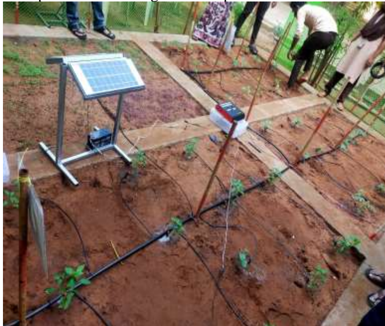
Fig.8. Real Time drip irrigation Implantation in Field
